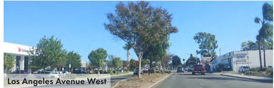
Figure 4.2: Existing Conditions Photos for Major Streets in Los Angeles Avenue Area.
