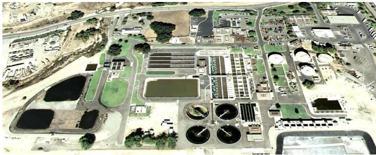
Simi Valley Water Quality Control Plant
