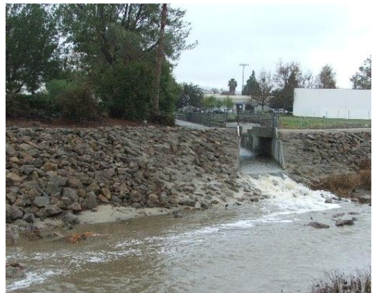
Storm drain channel
