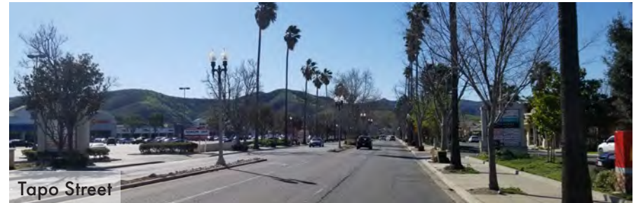
Figure 4.4: Existing Conditions Photos for Major Streets in Tapo Street Area.
