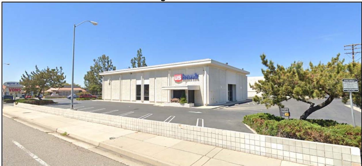
Existing Building from Los Angeles Avenue
