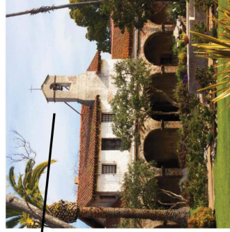
BELL TOWER EXTENDS ABOVE ROOF LINE IN MISSION STYLE ARCHITECTURE. HORIZONTAL BANDS OF MOLDING AT TOP AND BOTTOM OF OPENINGS REDUCE VERTICAL SCALE. BELL LOCATED IN THE TOWER IS NON-FUNCTIONING AND IS FOR AESTHETICS ONLY.
