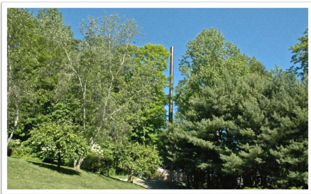
Desirable Monopole Design on Private Property
