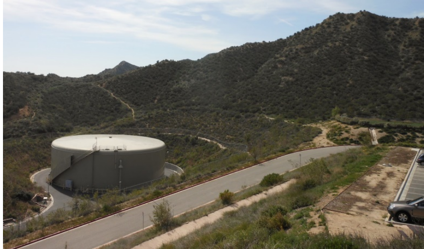
Typical Simi Valley Water Tank Site
