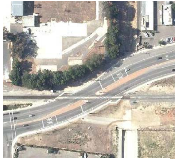
Figure 5-3: Los Angeles Ave.-Las Lajas Aerial Photograph
